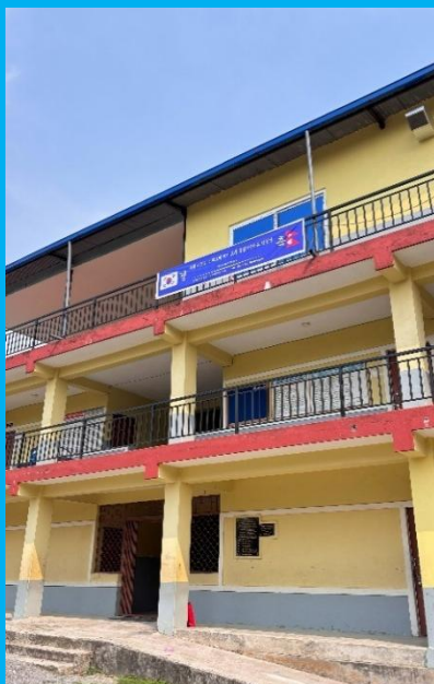
Construction for vocational class at Shree Saraswati Secondary School, Pokhara-33.
