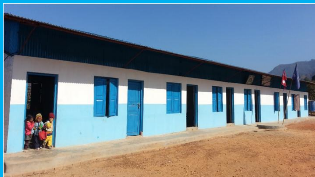
School building rebuilt at Shree Bagh Bhairab Primary School, Gorkha-02, following the 2015 earthquake.
