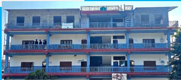
Construction for vocational class at Shree Janapriya Secondary School, Pokhara-8.
